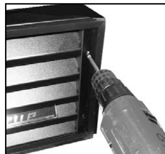
Image 3. Loosen but do not remove 4 Phillips screws inside the grill frame.
