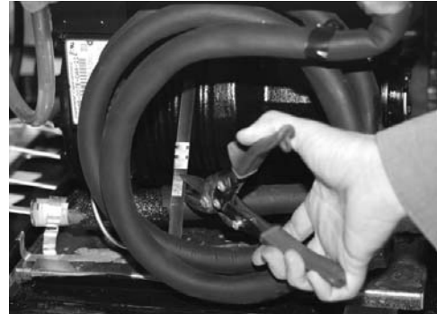
Cutting band around compressor
