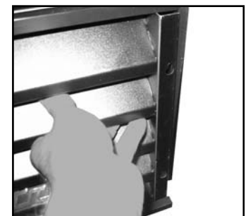
Image 4. Lift the grill up until it clears the screw key hole slots.
